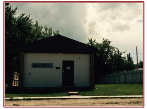
Sasktel Building, 1 st Street
