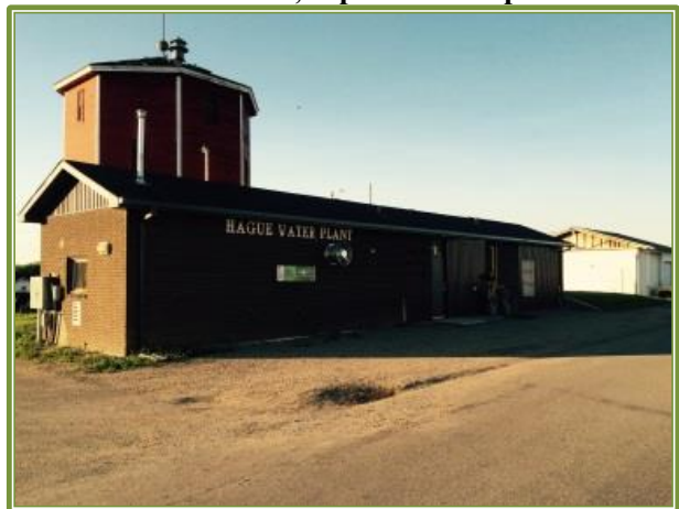
Water Treatment Plant, expansion completed in 2015
