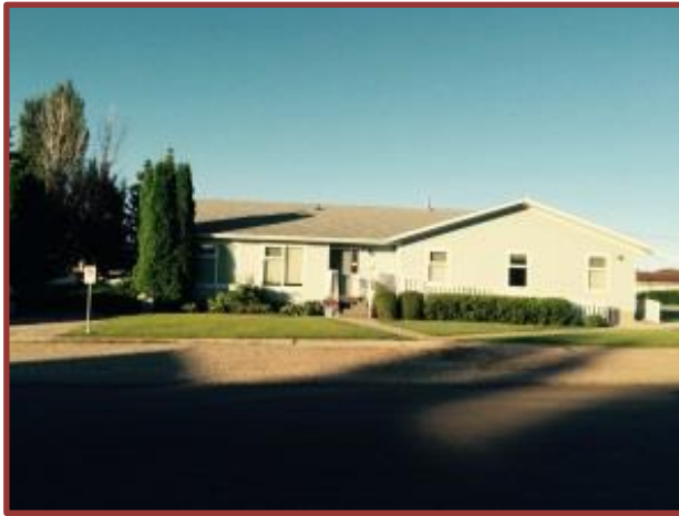
Sunshine Housing, 6 th Street
